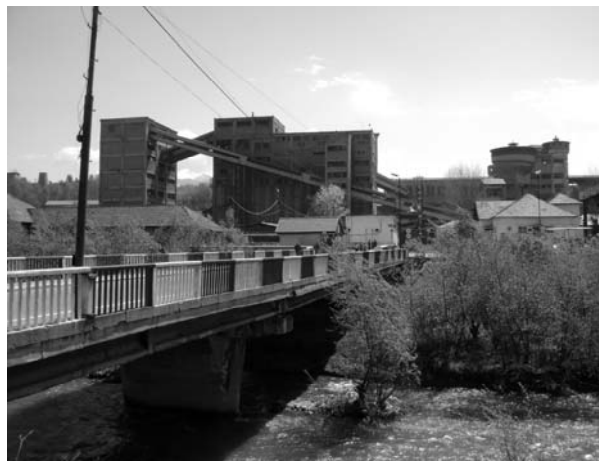
Photo 1. Petrila coal preparation plant
