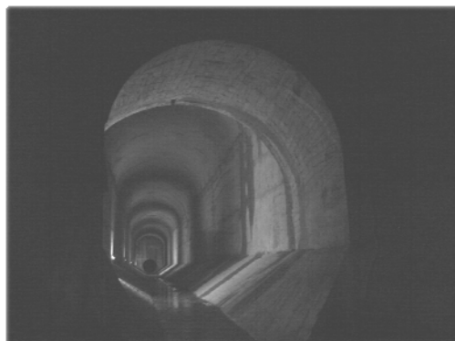
Fig.2. Settling underground reservoir Livezeni
